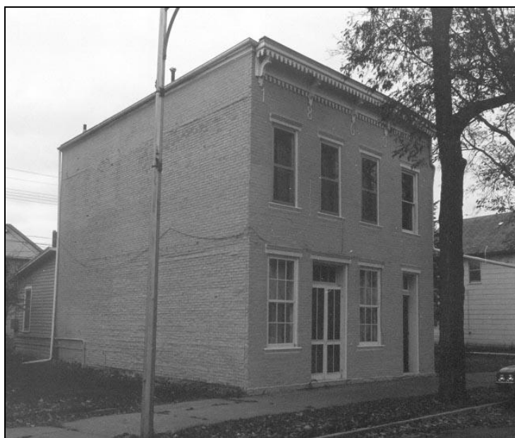
413 South First Street (1979 photo)
