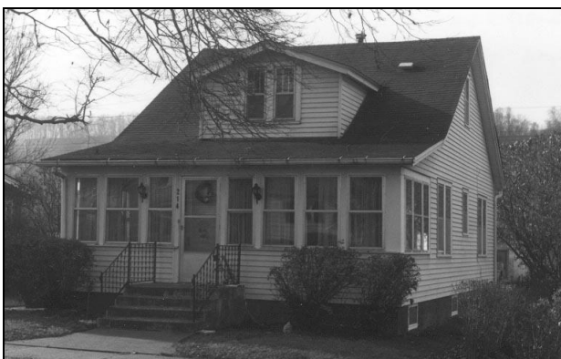
214 South Second Street (two-pitch front roof)
