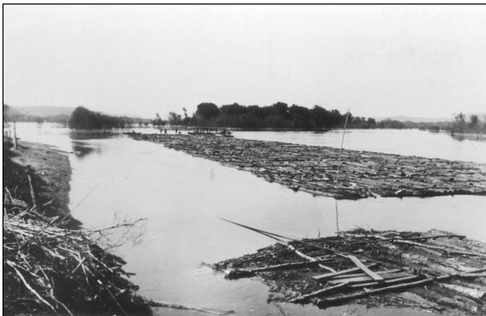
Willow mat base for a new wing dam
