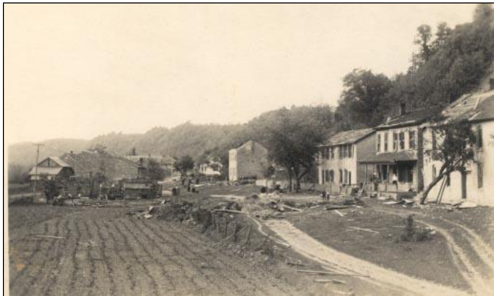
Tornado damage, May 21, 1918, view south
