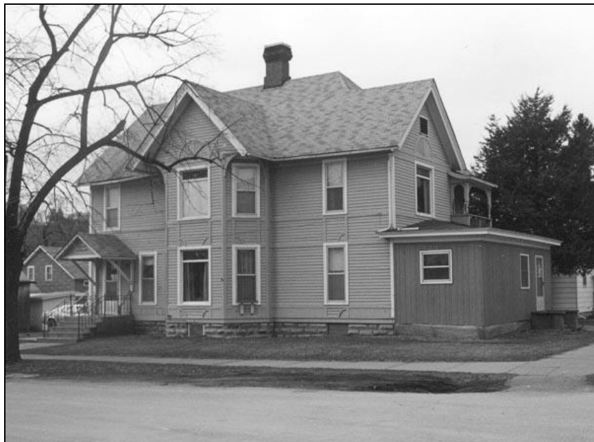
130 South River Park Drive (1979 photo)
