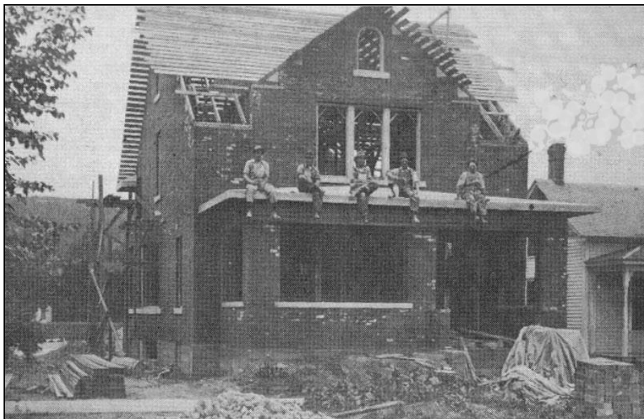
Ihm House, North River Park Drive, under construction, 1927 ( Press , March 5, 1927)
