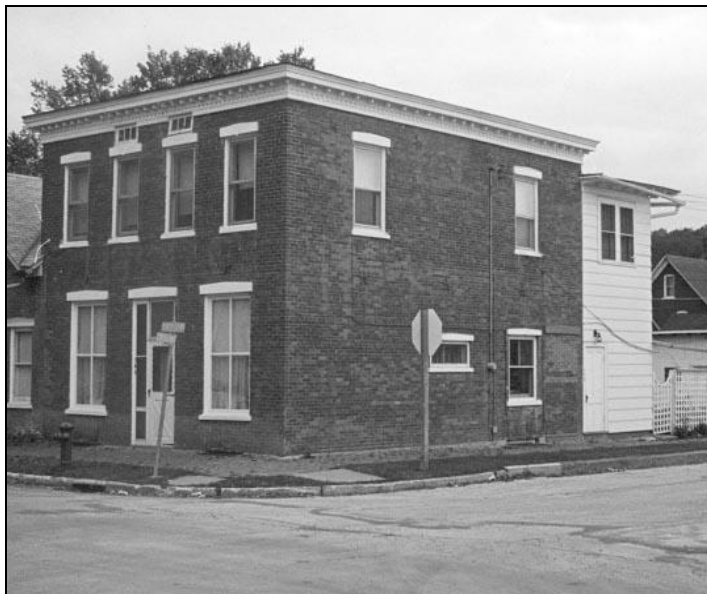
300 South First Street (1979 photo)
