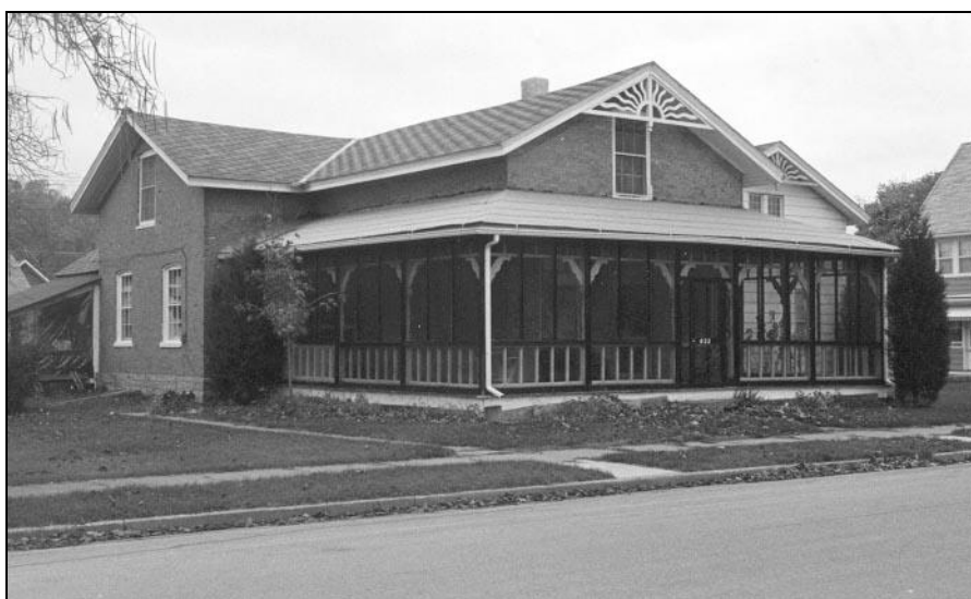
822 South River Park Drive (1979 photo)
