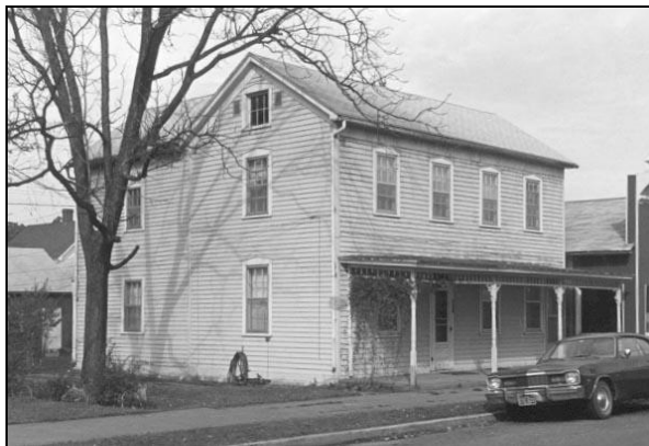
522 South First Street (I-house with rear wing)
