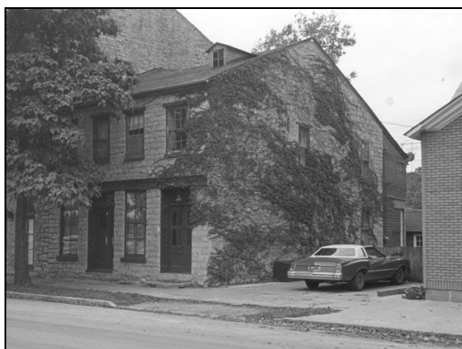
216 South River Park Drive (1979 photo)
