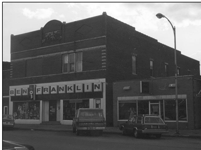
422 South River Park Drive (overall factory and twin storefronts)
