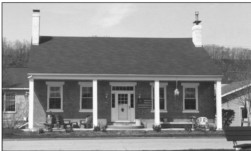
910 South River Park Drive (c.1856-62) National Register Listed
