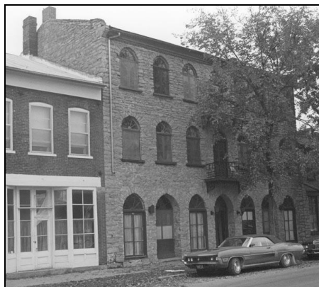
222 South River Park Drive (1979 photo)
