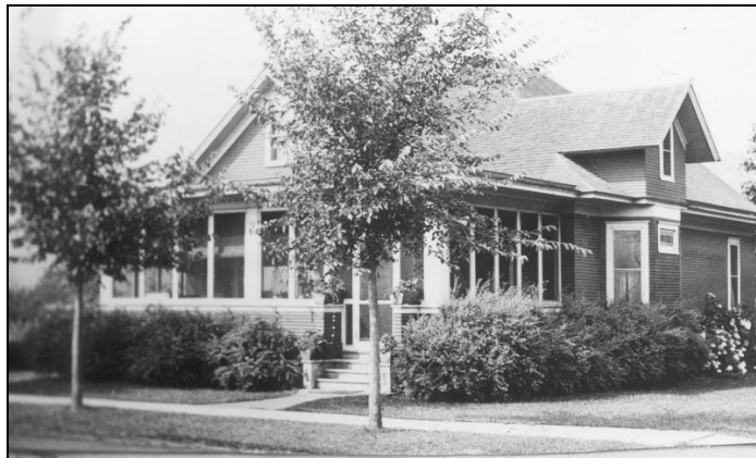
802 South River Park Drive (hip roof, original appearance)
