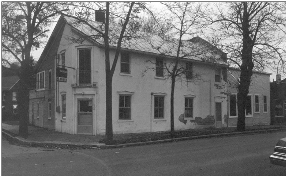
310 South First Street (1979 photo)
