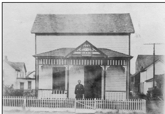
11 Wieland Street, original appearance
