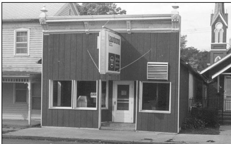
520 South First Street, rare metal cornice example
