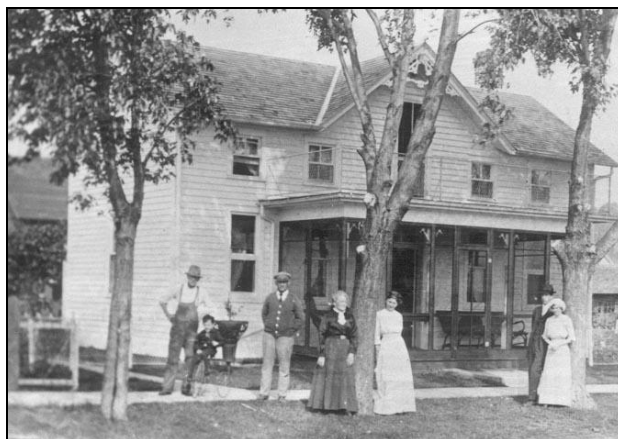
310 North River Park Drive (story-and-a-half I-House, non-extant)
