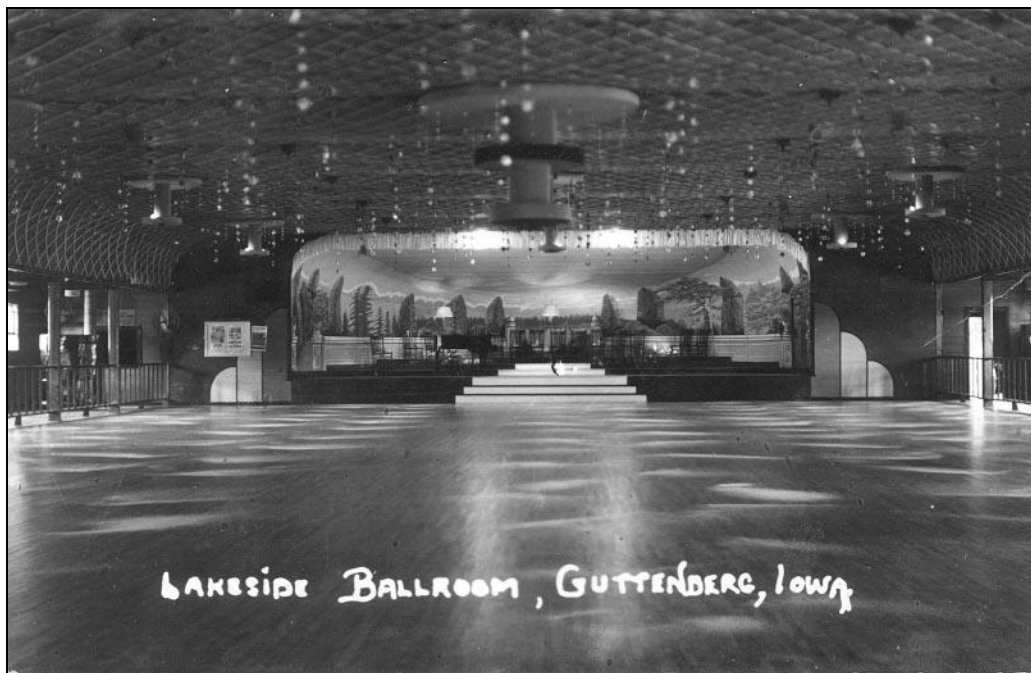
Lakeside Pavilion interior (courtesy of N. Thein)
